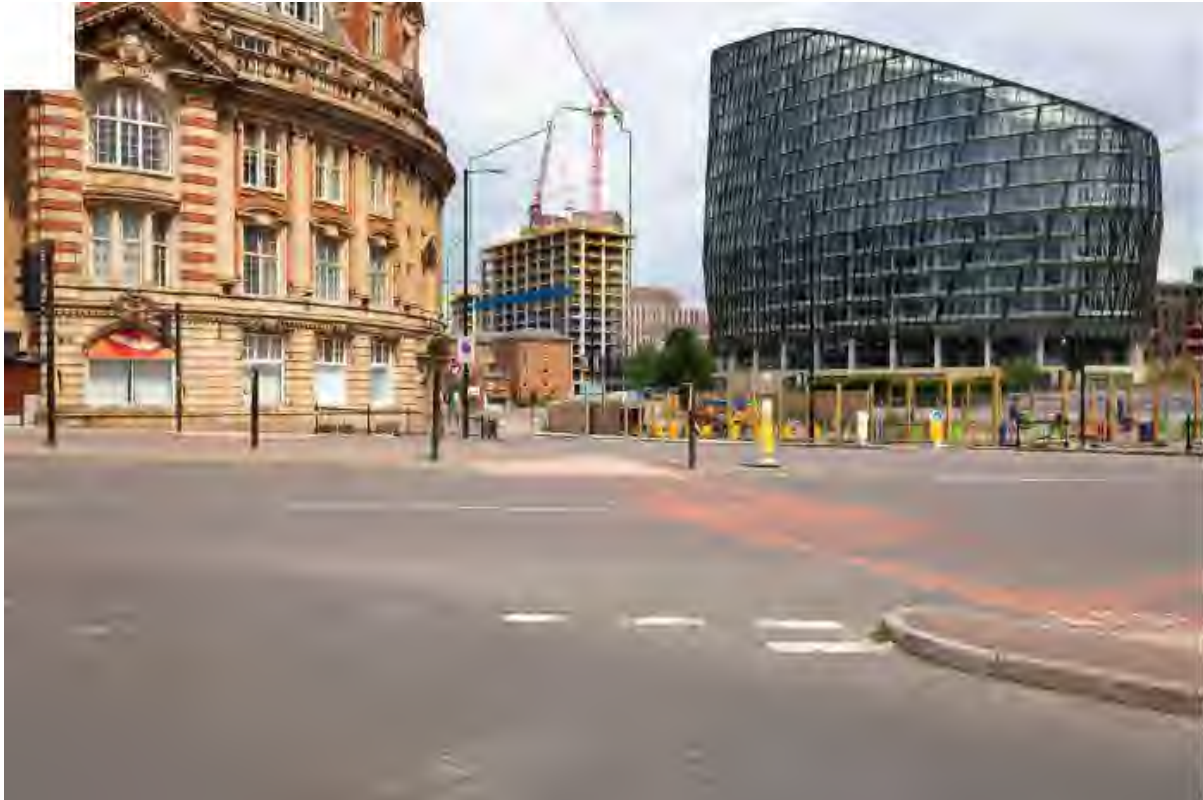
Viewpoint 9: View from the junction of Corporation Street/Miller Street (facing north east) (from Victoria Rail Station and setting of Grade II Parkers Hotel) (proposed)
